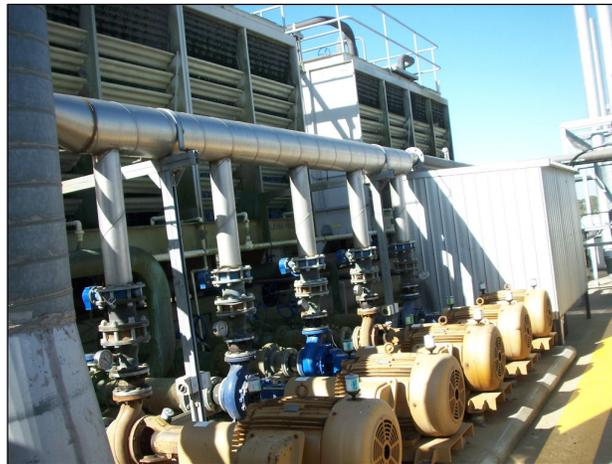
The system consists of five pumps and four cooling towers. The system had installed PLC control, however was bypassed as the control never worked successfully. At the outset of this project, therefore, the system was operated manually from summer to winter.
